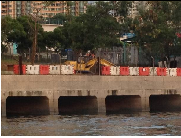
Photo 3.17 Backhoe for dredging/clearing mud/sludge over box culvert discharge point
