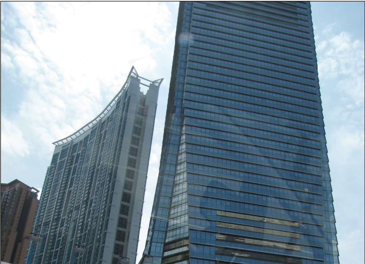
VSR 8 International Commerce Centre (ICC)
